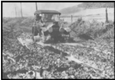
Hwy 101 before paving
